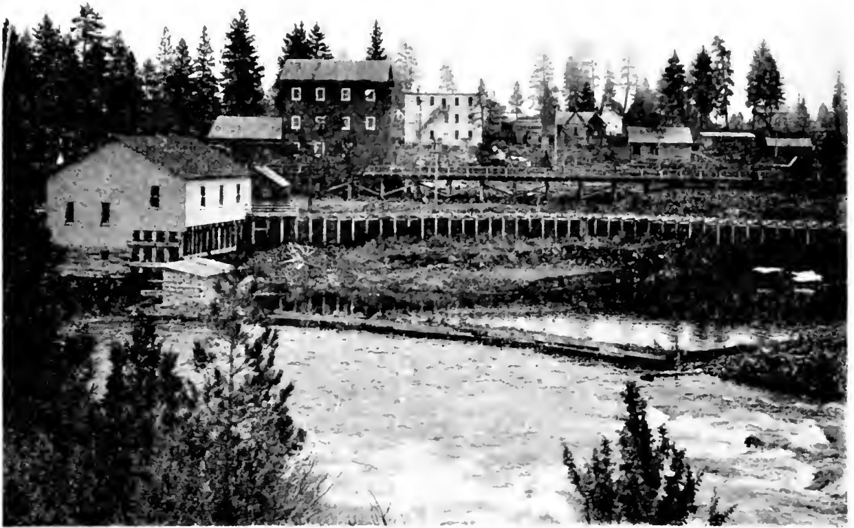
Bend Generating Station - constructed in 1910 by Bend Water, Light and Power Company.
